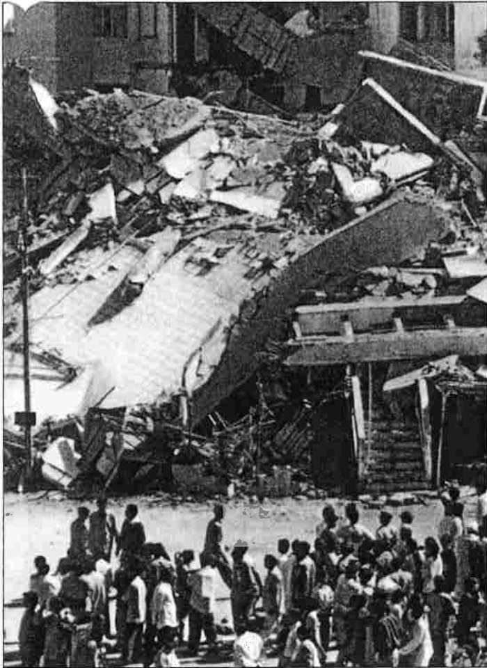
D Earthquake damage
