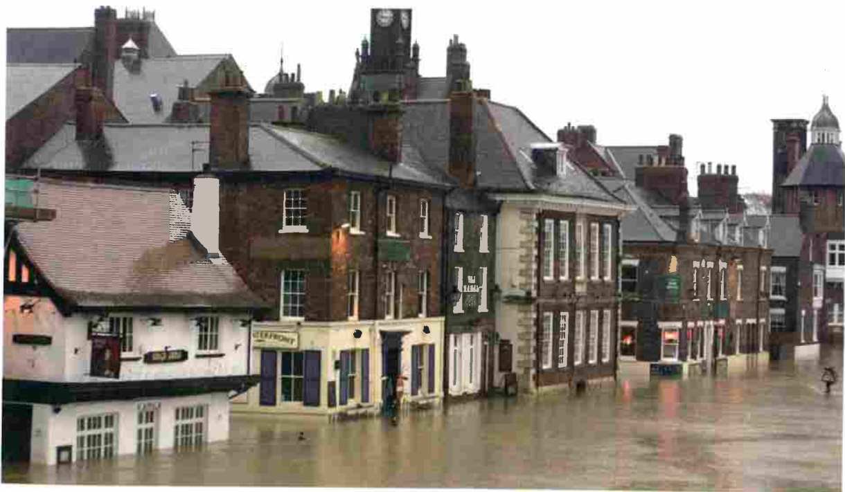
Figure 5.16 Flooding in York, 2000
